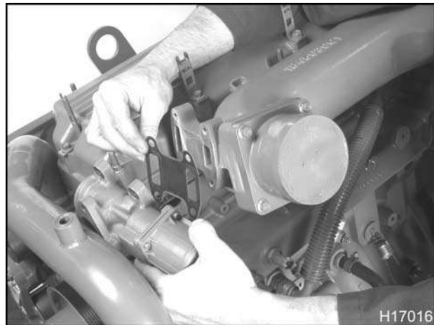
Figure 94 Removing the EGR valve to EGR mixer gasket
