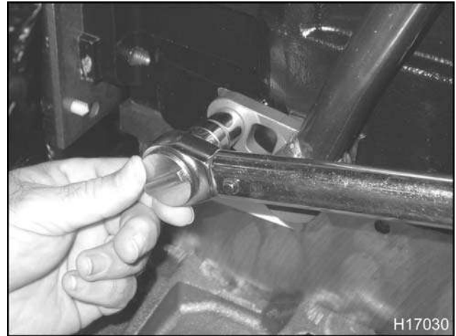
Figure 124 Torquing the EGR cooler return tube mounting bolt
