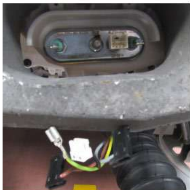
Remove the heater sockets
