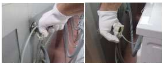
Turn off the tap and disconnect the hose from the valve
