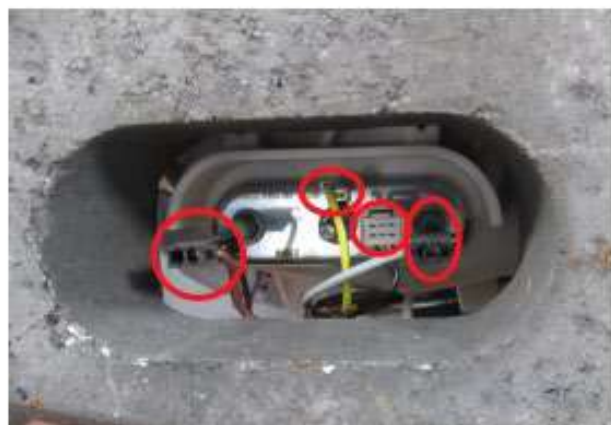
Remove the heater sockets
