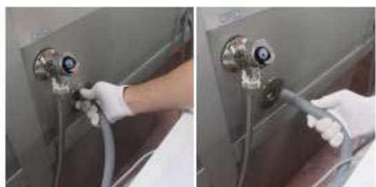
Disconnect the drain hose
